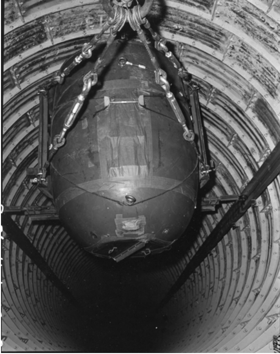
PLK 46-3 8Feb55 – ESS weapon being lowered in shaft.
